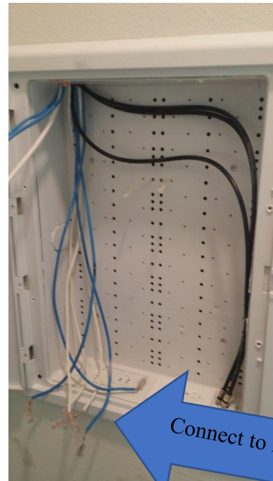
APARTMENT WIRING PANEL – FOUND IN A BEDROOM CLOSET.
